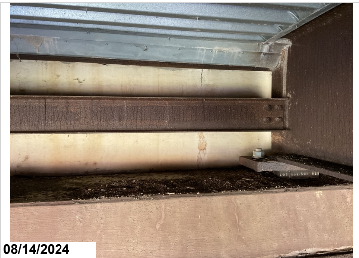
Bent 4 abutment, Cracking in backwall, CS2
