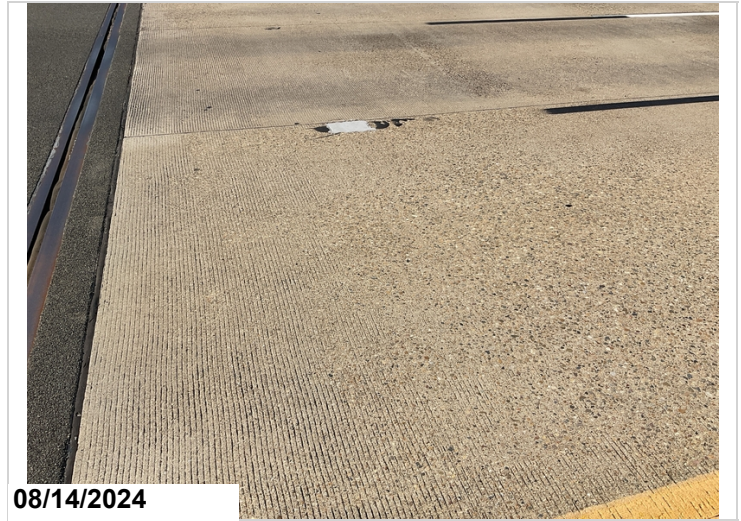
Beginning of bridge approach slab, Patched area, CS2
