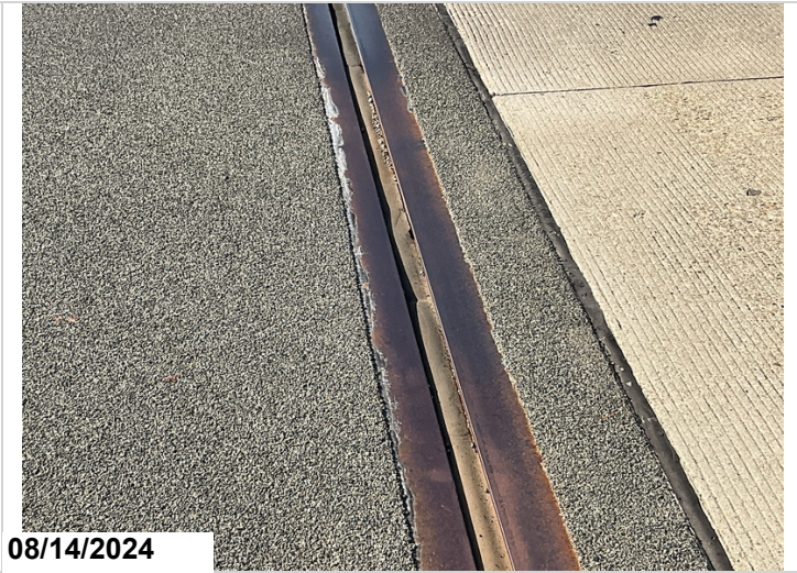
Beginning of bridge, Joint damage, CS3
