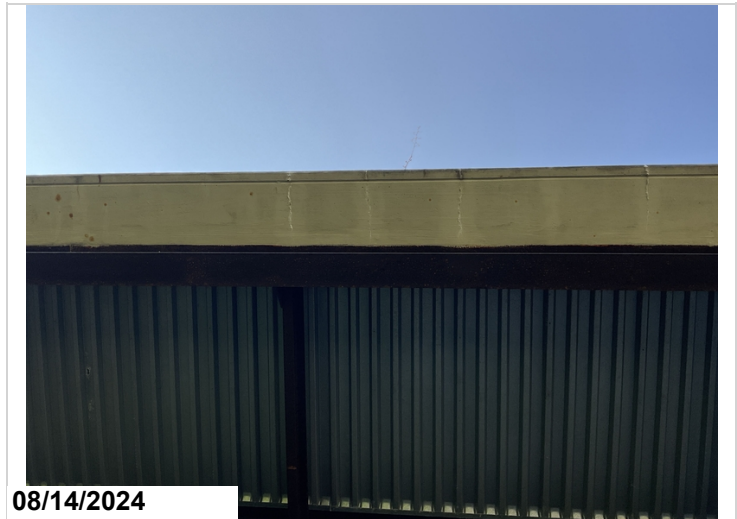
Deck, Undersurface, Efflorescence is present in various locations on both right and left overhangs, CS2
