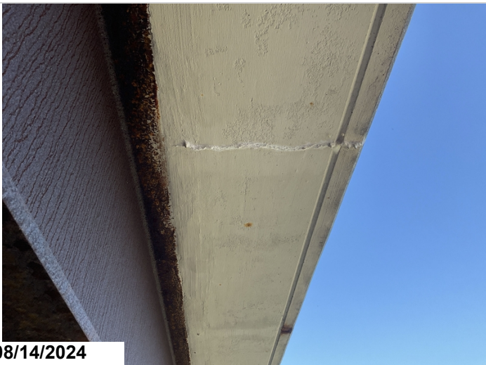
Deck, Undersurface, Efflorescence is present in various locations on both right and left overhangs, CS2
