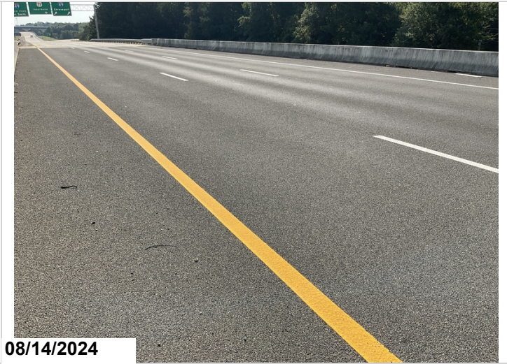
Polymer wearing surface photo
