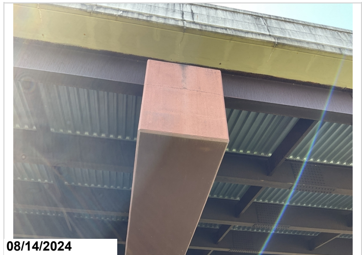
Bents 2 and 3 caps, Various locations of cracking, CS2
