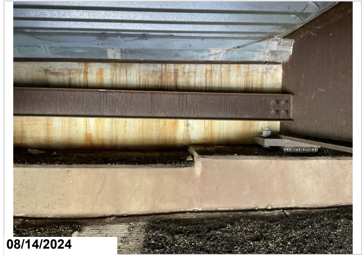
Bent 1 abutment, Cracking in backwall, CS2
