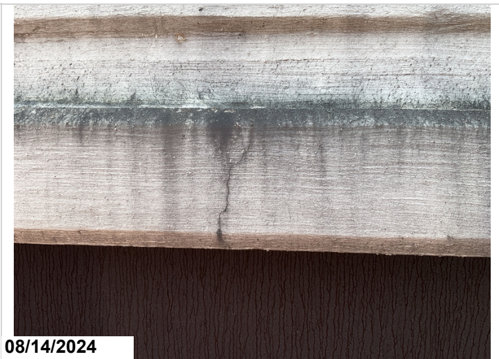
Concrete bridge railing, Cracking on both right and left sides, CS2
